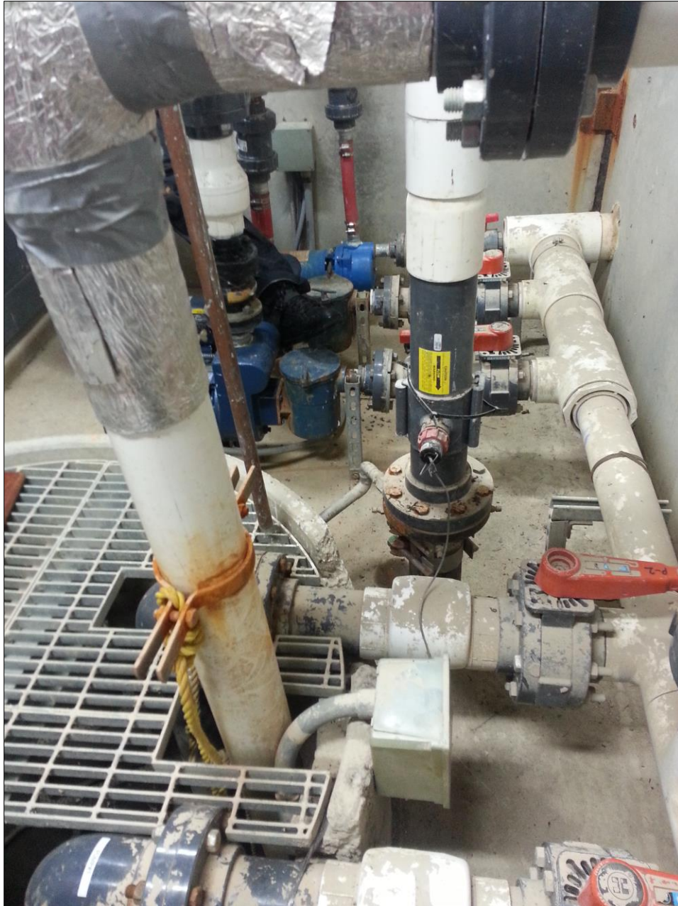
Figure 4-2. Surface Water Pumps – Note Silt from Flooding on Pipes
