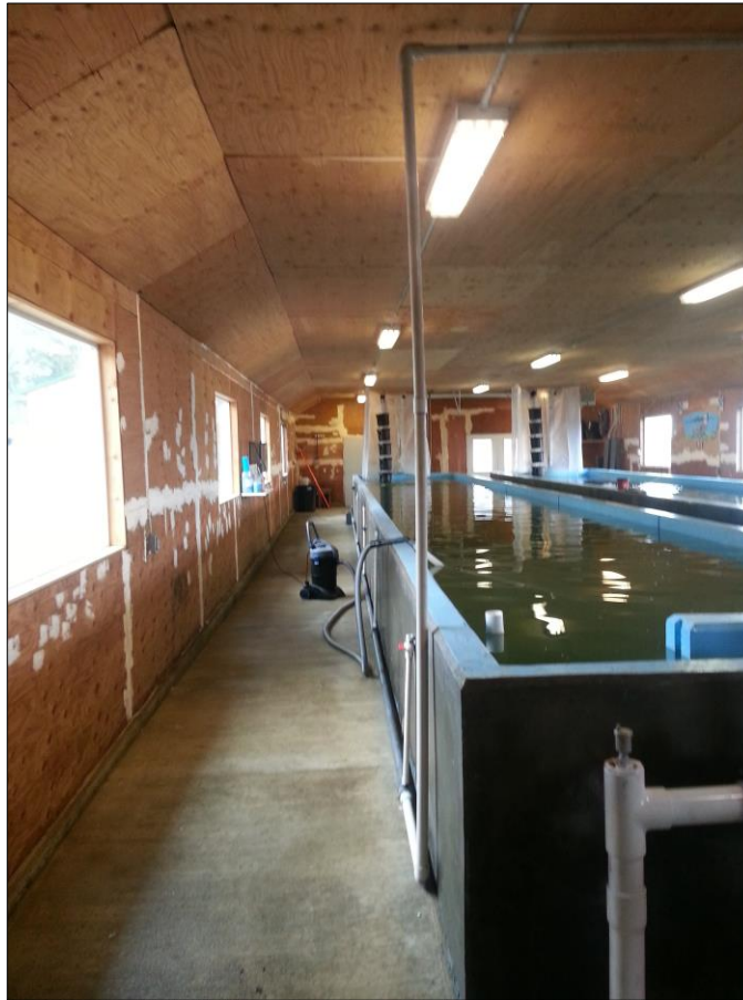
Figure 4-7. Lower Hatchery Building Raceways
