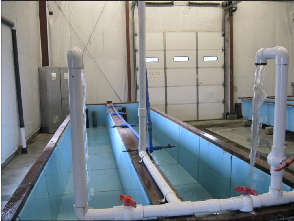
Figure 4-5. Upper Hatchery Building Fiberglass Troughs, Water and Air Supply Piping
