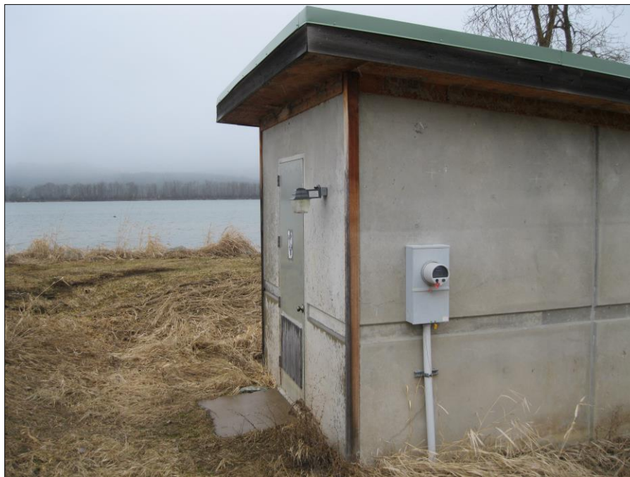
Figure 4-1. Surface Water Pumpstation – Note High Water Mark on Wall Above Meter
